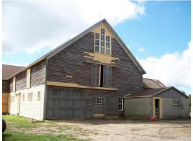
A before shot of a barn at Cherry Hill Farms in Ludington, Mich., left, is transformed with a little paint by Tim and Christine Barnes of Barn Painting and Advertising in Adams County. (Submitted)
